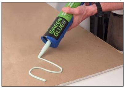
Green Glue can be used to soundproof walls, floors and ceilings. It can be used both in new construction, building upgrades and renovations.
